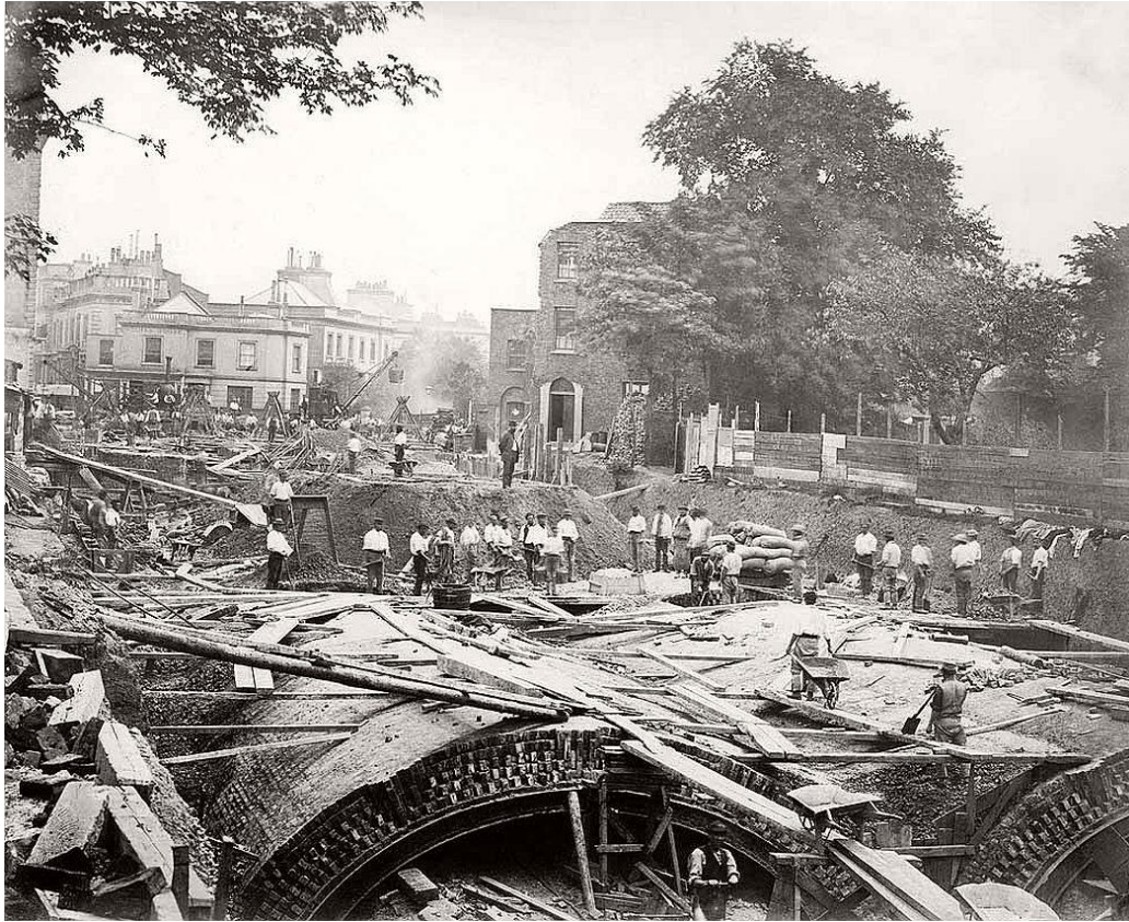
London Underground Construction (Victorian Era). Construction work near South Kensington Station
