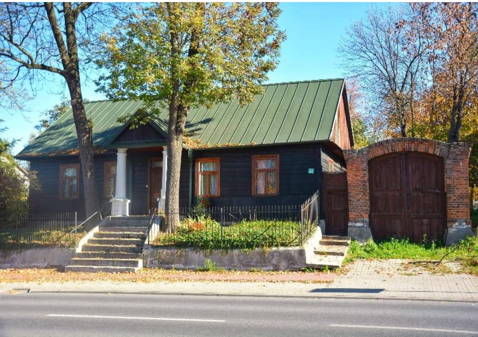
Historical masonry building in Głusk
