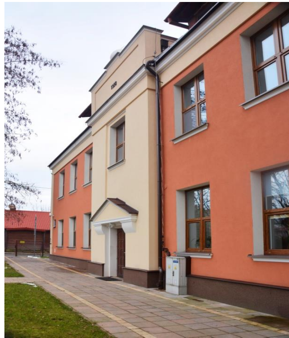
School building at Zdrowa St
