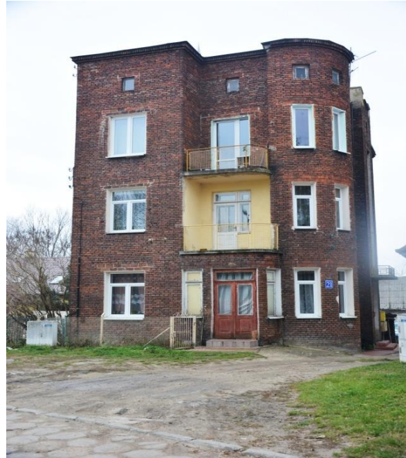
Masonry town house at Handlowa St 21
