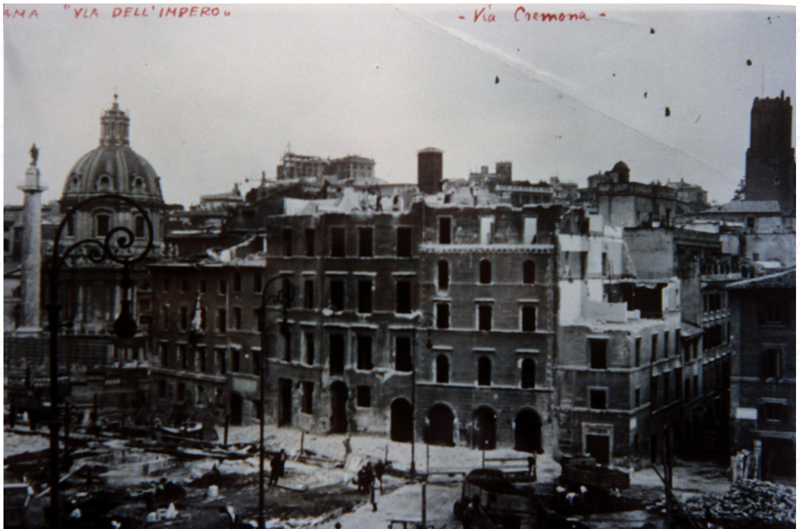
Rome, Via dei Fori Imperiali during the demolition of the district and opening the new street (C. Bellanca 2003).
