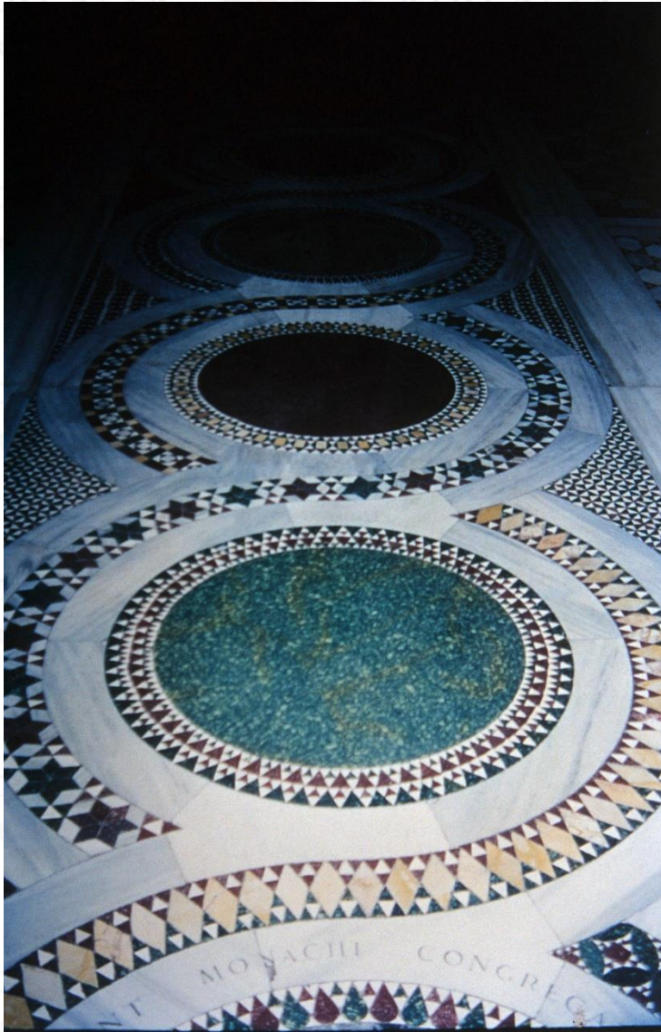
Rome, Church of St. Prassede, new pavement with the insertion of ancient marble. (CB 1994)
