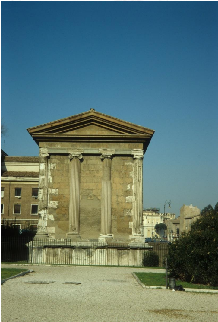
Rome, Tempio di Portuno after restoration by Antonio Muñoz
