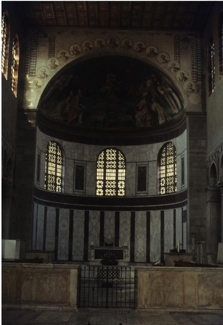
Santa Sabina, apsis after restoration work by Muñoz (CB. 1994)
