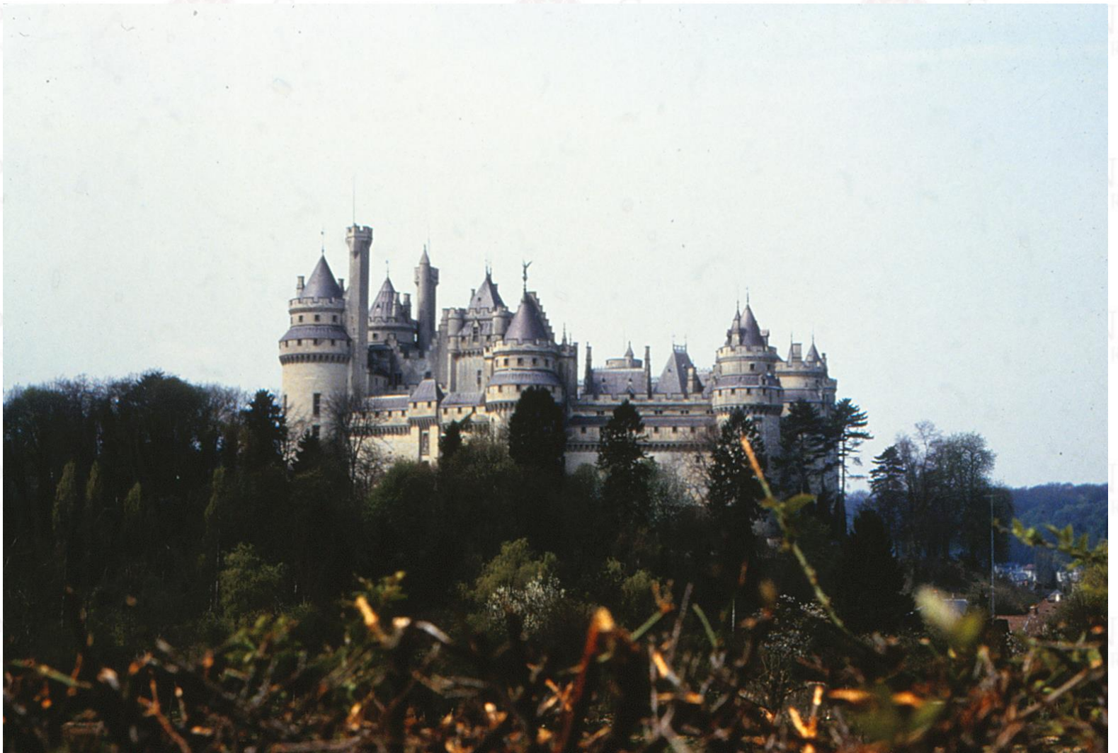
Pierrefonds, general view (CB 1987)
