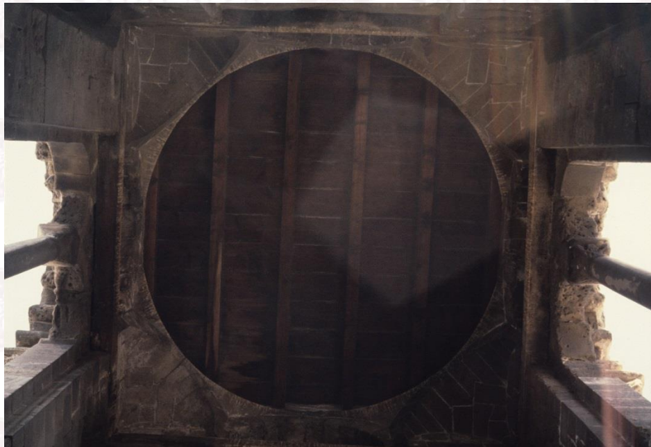
Detail of tower bell ceiling (photo by CB, 1984).
