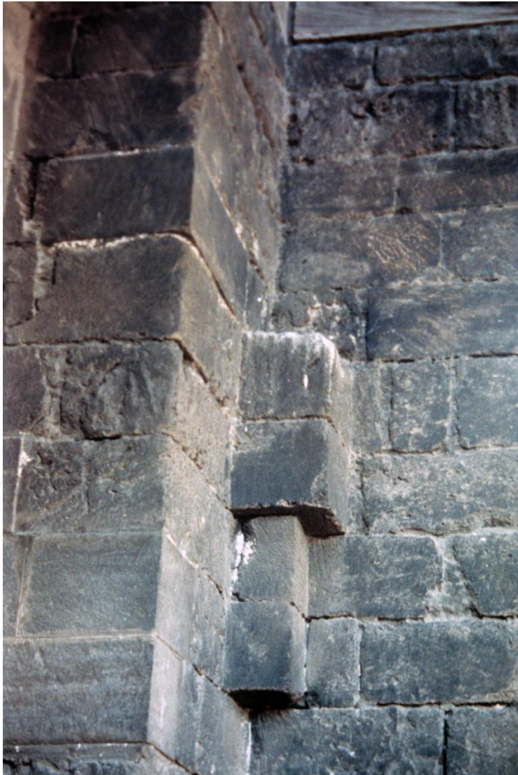
The vault of first level (photo by CB, 1984).
