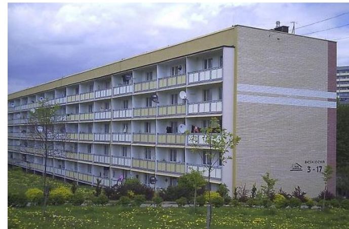
Block in Jastrzębie-Zdrój, in the construction of which the "Fadom" system was used. [4]
