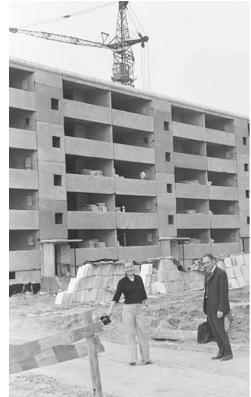
Building assembly in the OW-T system. [5]
