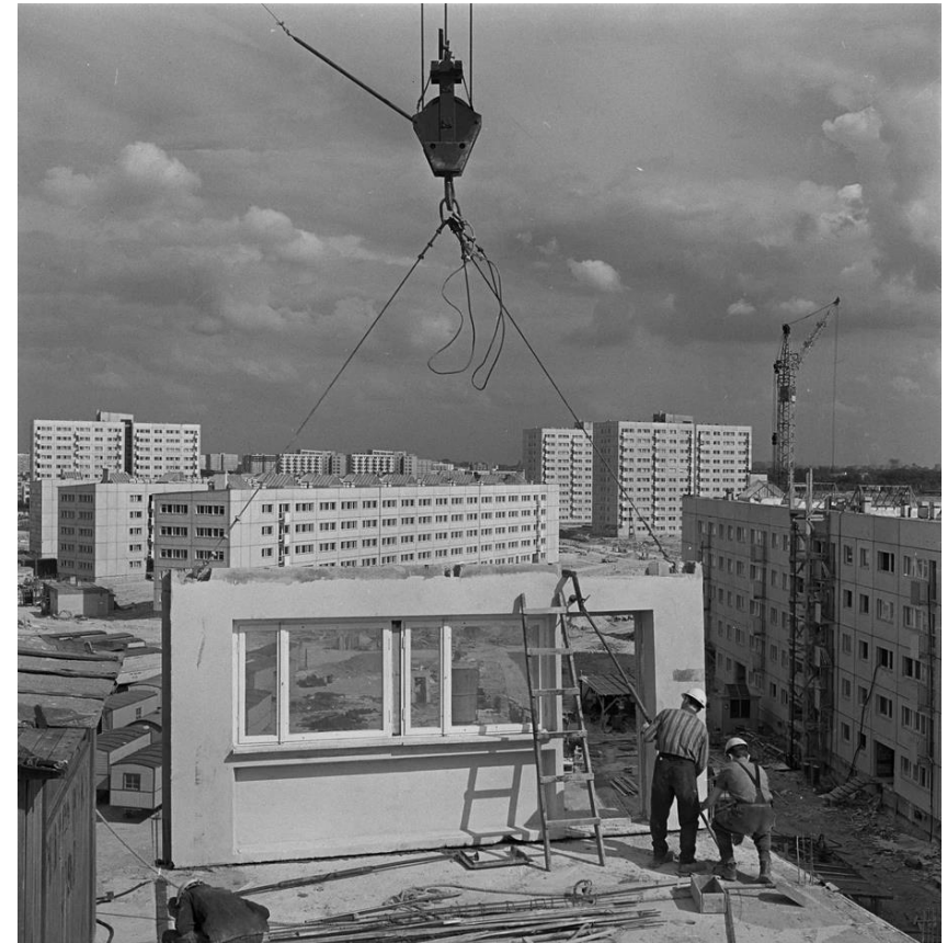
Construction of a housing estate using large-panel technology. [15]
