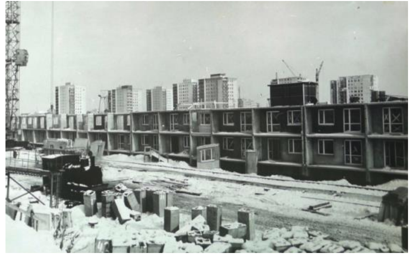
Construction of blocks in the "Fadom" system in the early 70s [13]
