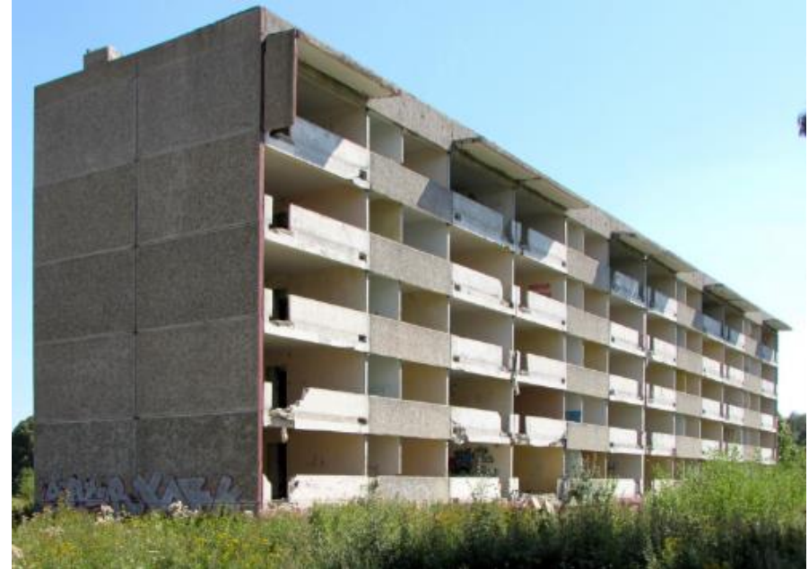
Abandoned block of flats from a large "Leningrad" type plate in Kłomina. [17]
