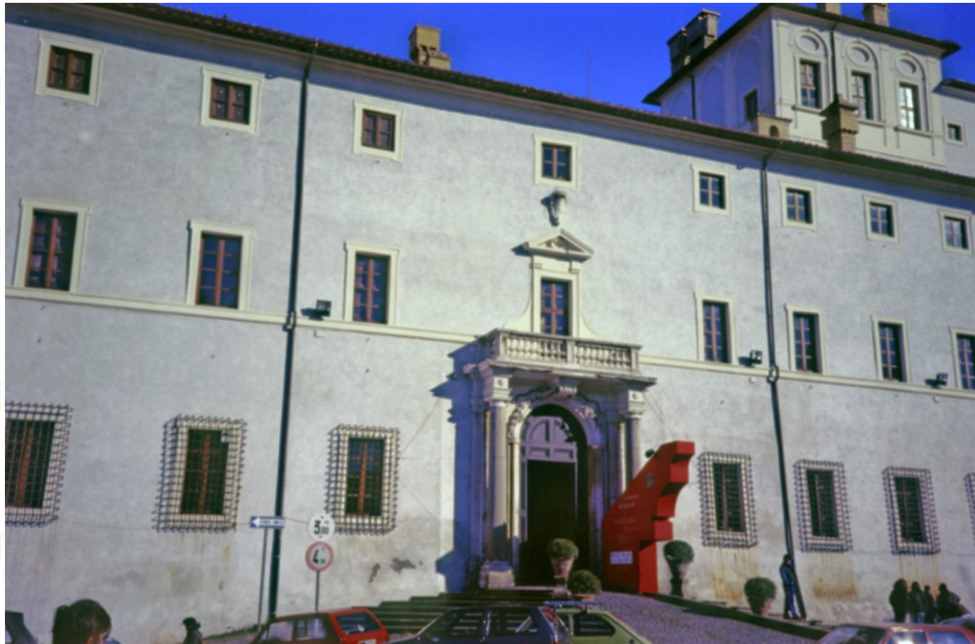
Ariccia, after the restoration with the “air colour”. (CB 1998)
