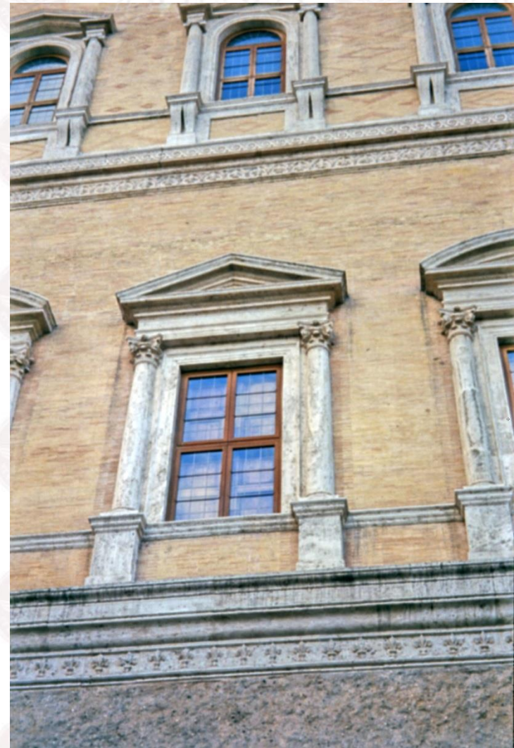
Roma, Palazzo Farnese; façades cleaning with different treatments according to the materials. (CB 1999)
