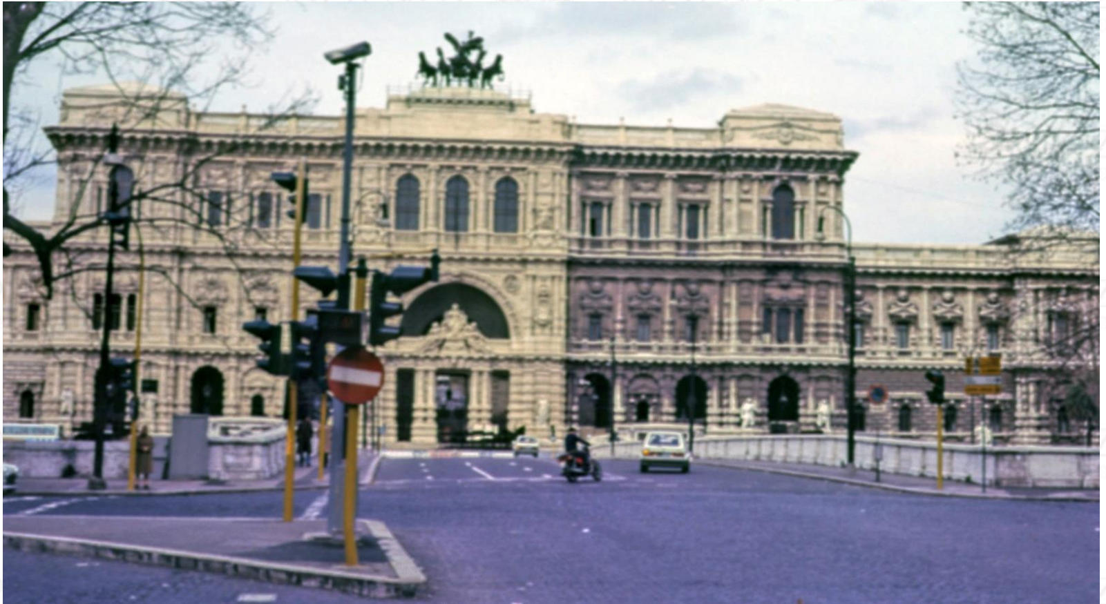
Roma, Palazzo di Giustizia, the cleaning during working progress. (CB 1983)
