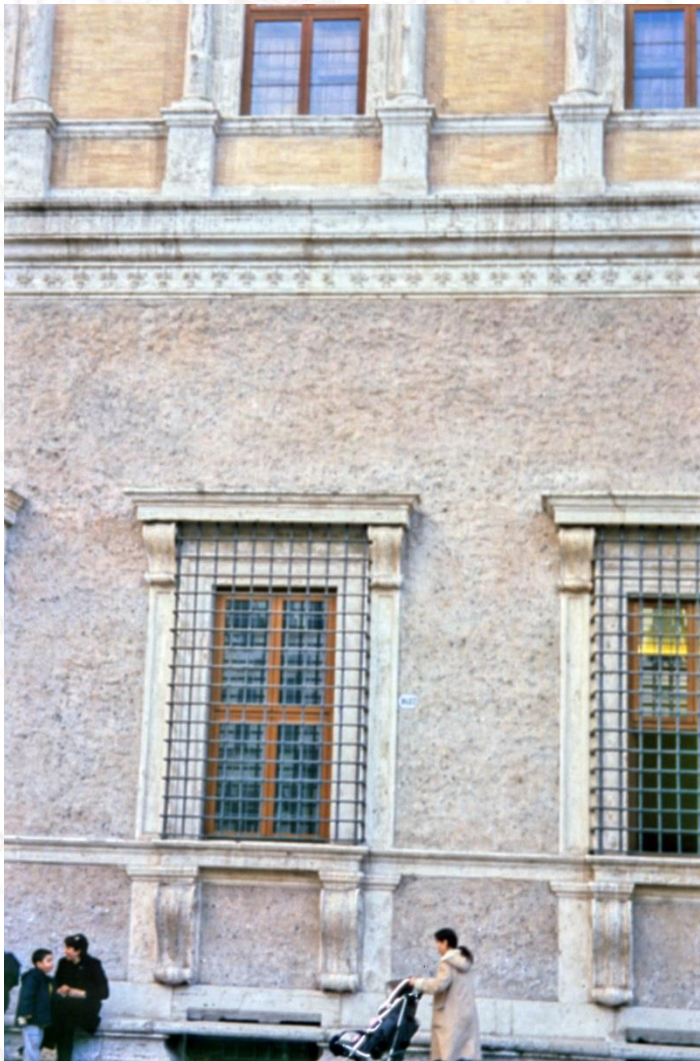
Roma, Palazzo Farnese; façades cleaning with different treatments according to the materials. (CB 1999)
