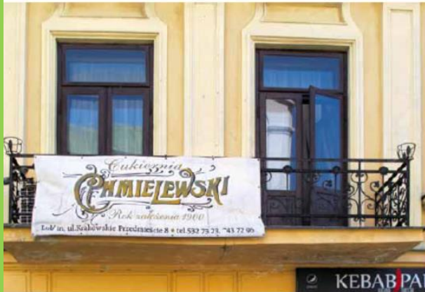
SIGNBOARD FIXED TO BALUSTRADE
