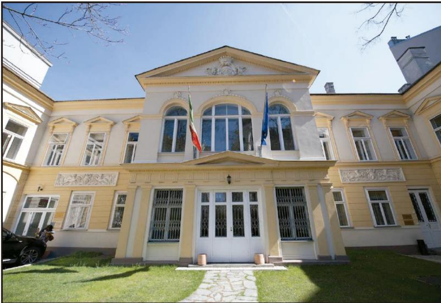
Façade after the restoration of 2014/2015. Photo by C.B. 2015
