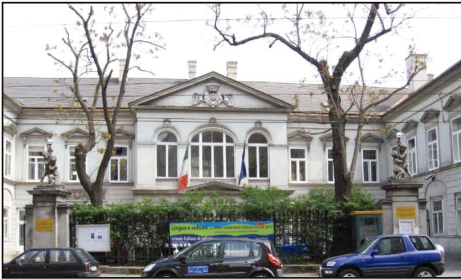
Palazzo Sternberg façade, before the restoration. Photo by C.B. 2012
