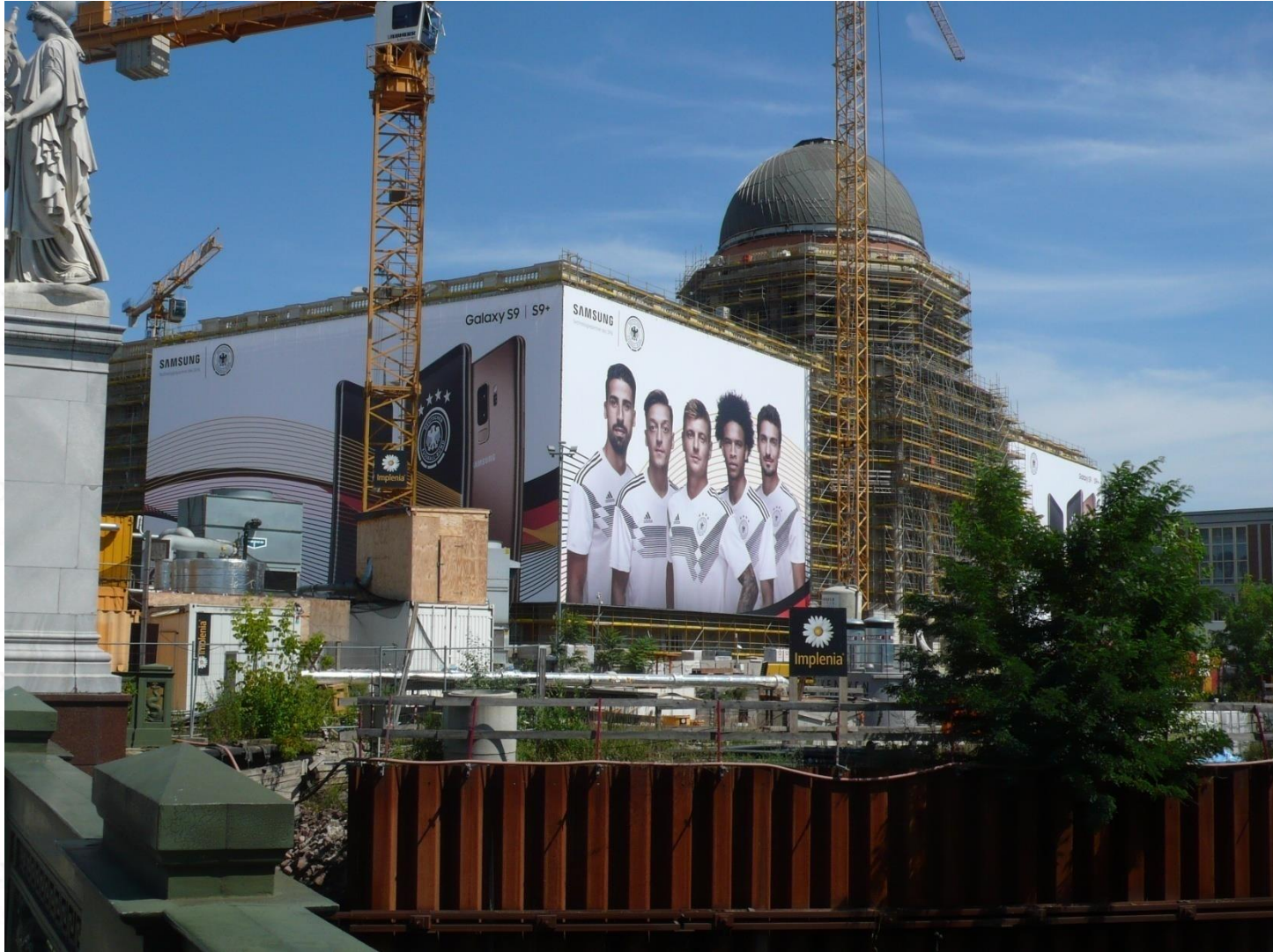
The construction site for the reconstruction of the Royal Palace (CB 2018)
