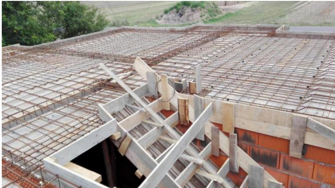
Fig. Monolithic reinforced concrete ceiling in progress [6].
