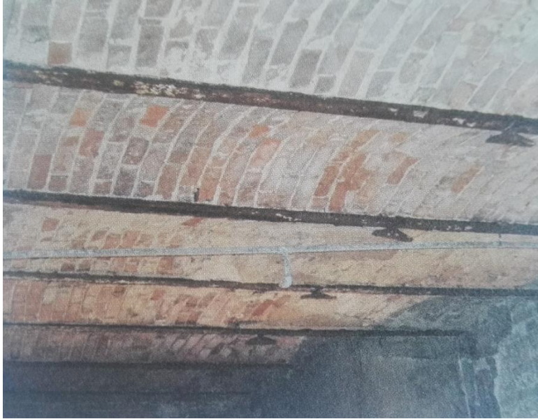
View of the segmental ceiling [4]
