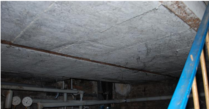
Renovated Klein ceiling in a historic building
