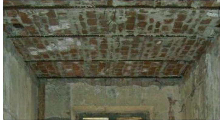
Klein's ceiling from underneath [6]
