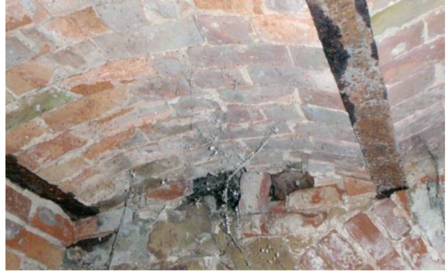
Segment ceiling from around 1908 [6]
