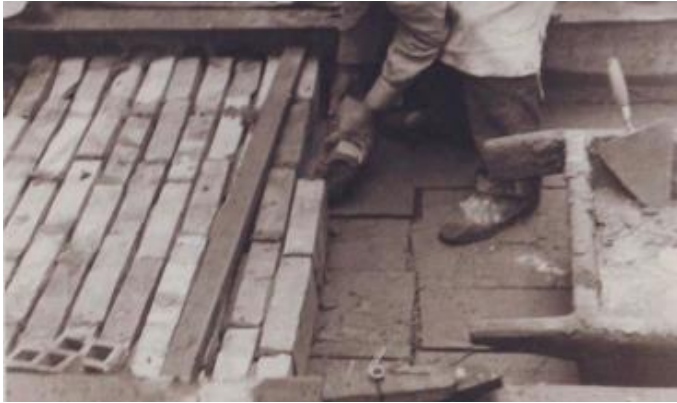
Making the Klein ceiling around 1928 [6]
