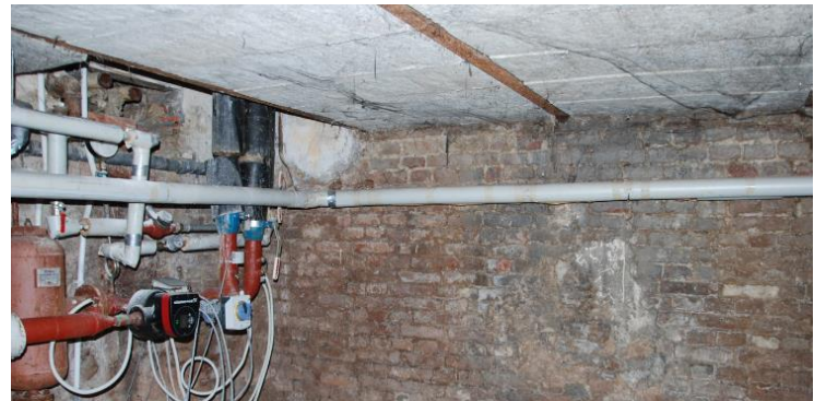
Renovated Klein ceiling in a historic building
