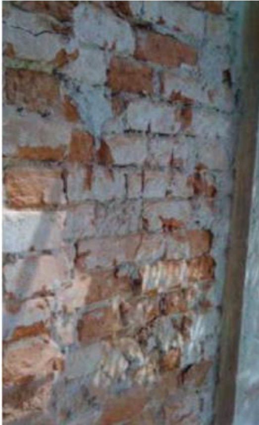
Destruction of the brick wall due to the use of cement-based plaster. [2]
