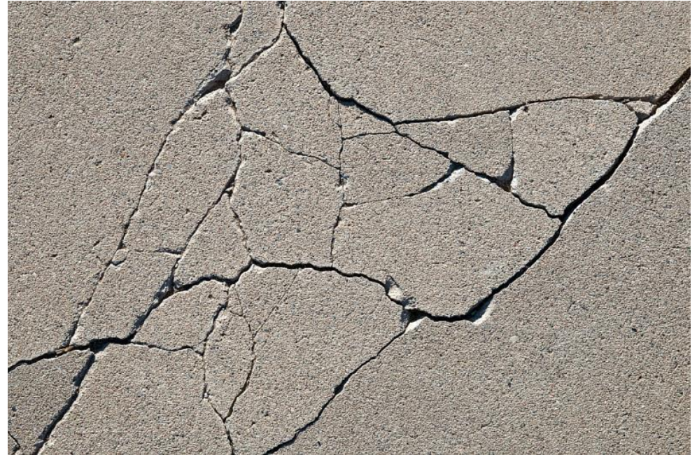
Cracking of the wall surface. [4]
