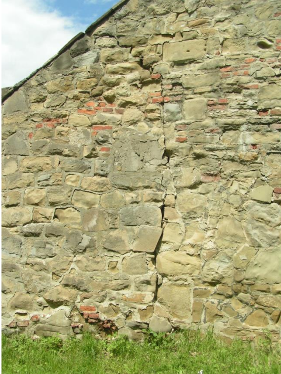
Vertical scratches in the wall. [3]
