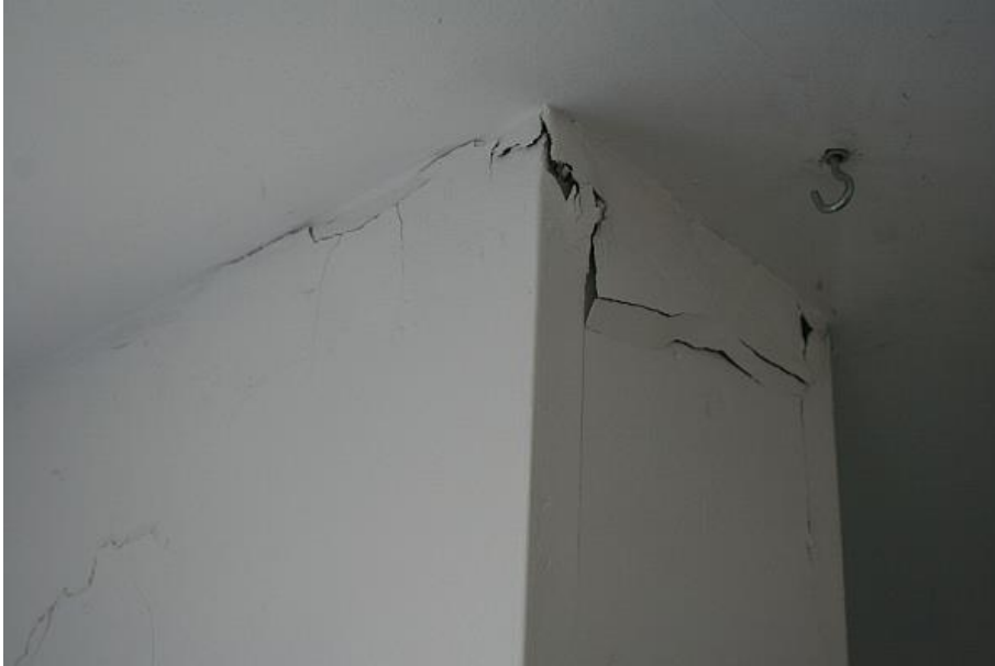
Cracks when connecting the wall with the ceiling. [4]
