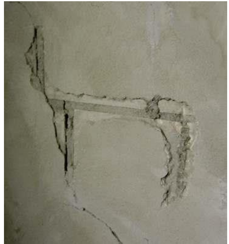
Open-cast of the plaster near the lynx - bad binding of wall elements. [4]
