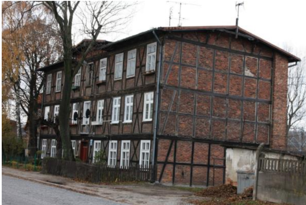
Historic tenement house ul. Sandomierska 49 in Gdańsk - half-timbered construction with a Prussian wall. photo: aspirin, source: http://zabytki.ocalicodzapomnienia.eu
