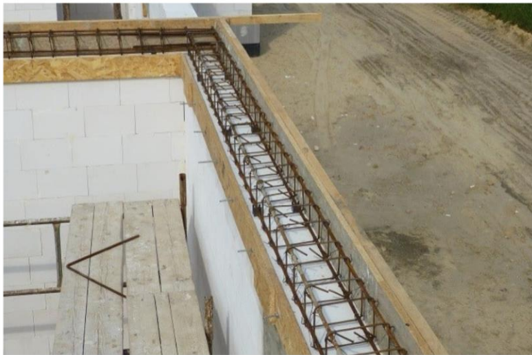
A tie beam with a prefabricated ceiling.
