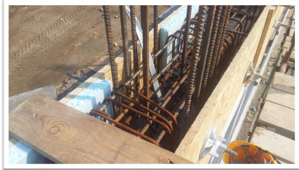
Reinforcement of the tie beam through a pillar.
