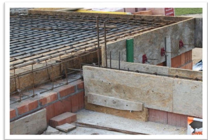
Fig. Prepared formwork for the rim and monolithic ceiling [3]
