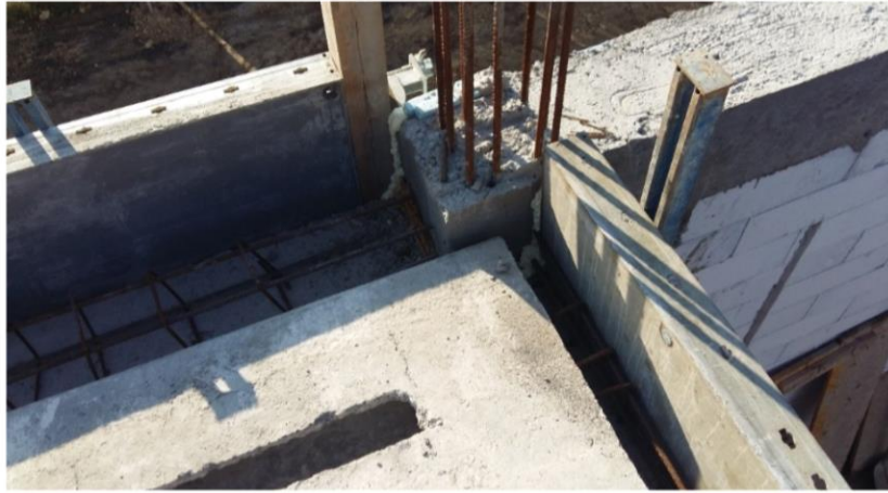
A tie beam with a prefabricated ceiling.
