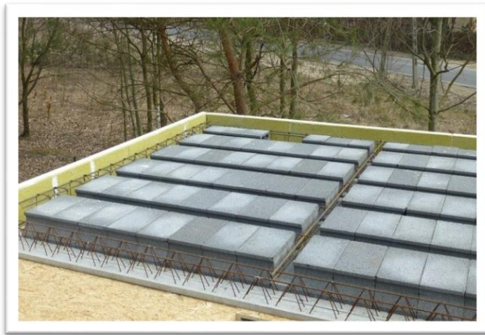
Fig. Ceiling coarse slab with finished wreath reinforcement [2]
