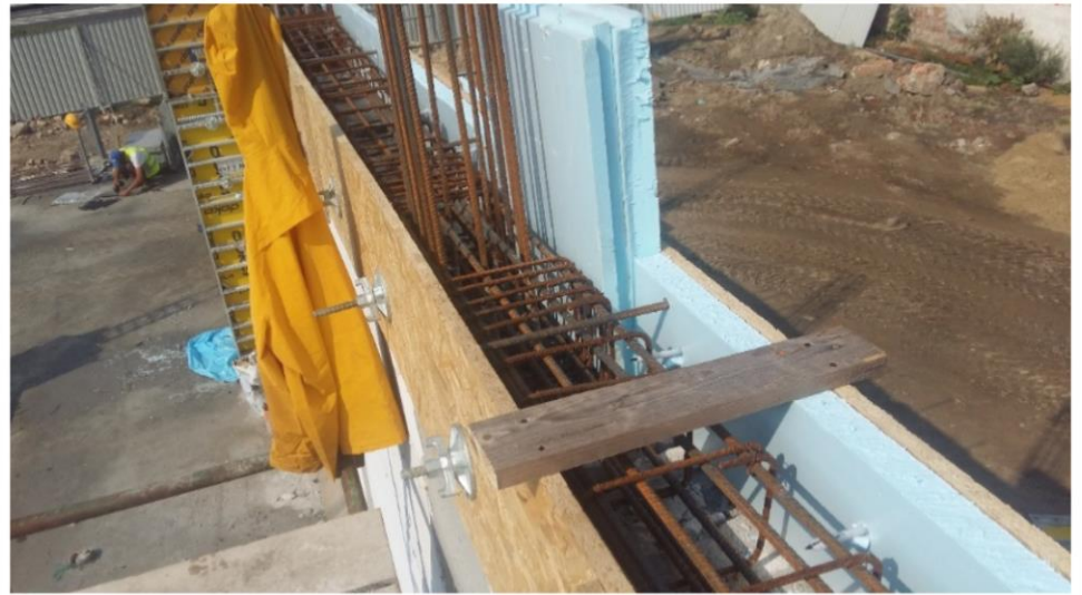
A tie beam made on the first layer of a brick wall with visible thermal insulation.
