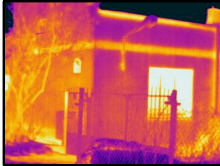
Thermal bridge on the rim [5]
