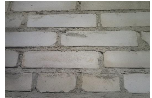
Fig. Brick wall. [2]
