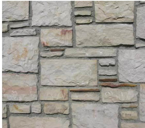
Fig. Example of squared wall. [2]
