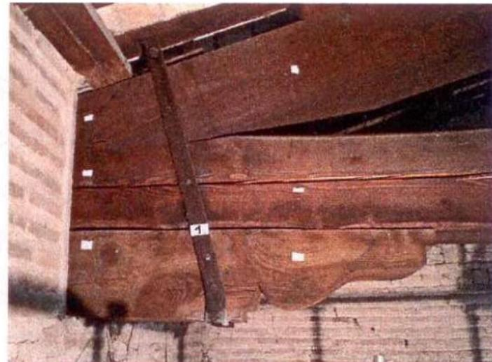
Moisture survey (left) and example of the coding assigned to the truss head with indication of the execution points (right).
