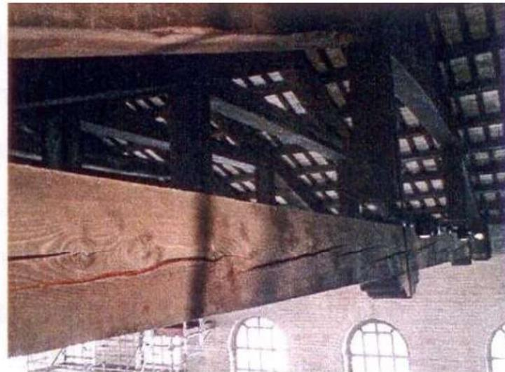
Vertical deviation between bracket and tie-beam (left) and longitudinal fissures due to tie-beam shrinkage (right).
