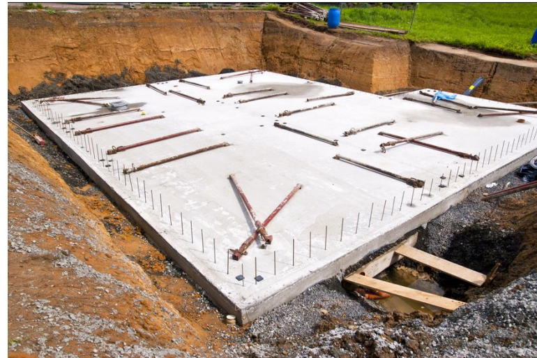
Photo. Reinforced concrete foundation plate [6]
