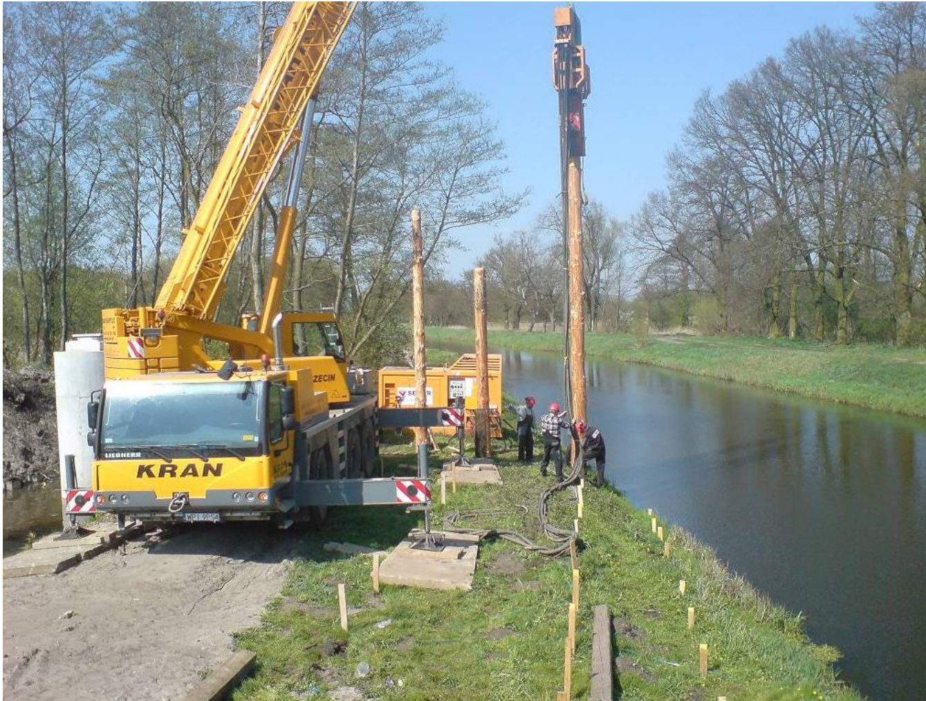
Photo. The process of introducing wood piles into the soil by vibrating [6]
