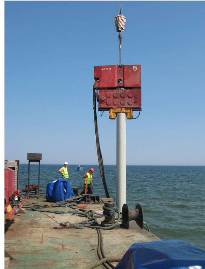
Photo. The process of introducing steel piles for the construction of a fishing pier [6]
