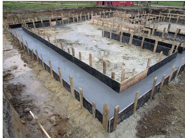
Fig. Reinforced concrete footbridges with formwork [6]
