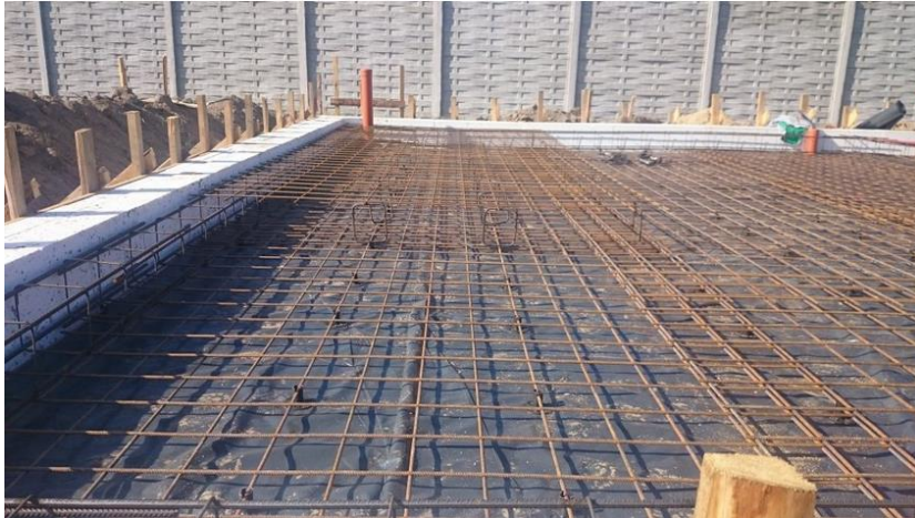
Photo. Reinforcement of the foundation plate [6]
