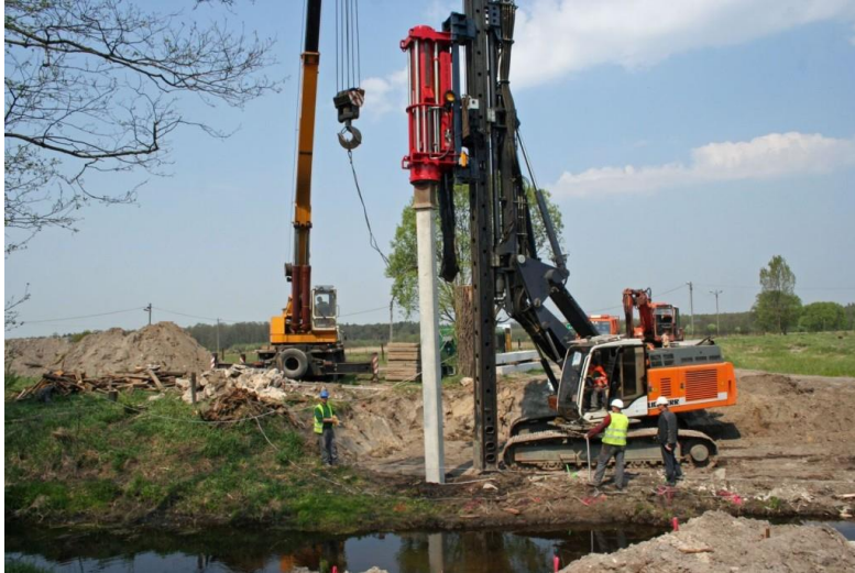
Photo. Introducing reinforced concrete piles into the ground by driving technique [6]
