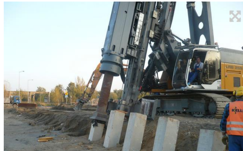
Photo.14 Placing piles in the ground by pressing [6]
